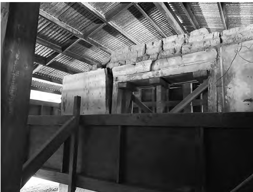
Bedroom wall showing original adobe bricks.
